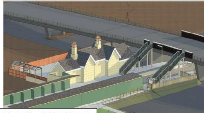
Existing View behind platform 2
